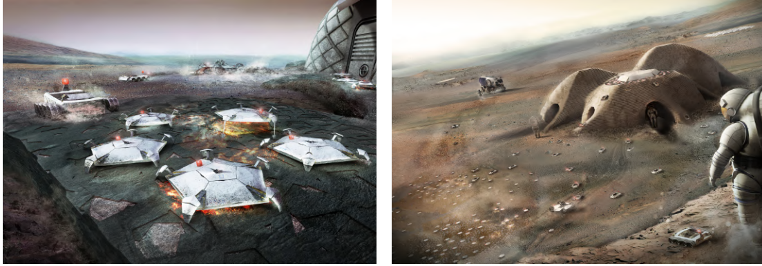
(a) Deposition and sintering of regolith layers by multiple RAC-T and RAC-M robots (b) Operational occupied outpost with continuous repair and infrastructure construction
