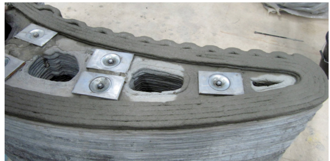
Figure 3: Internal structure including functional voids and reinforcement. The rectangular shaped steel plates are the customised washers for threaded rebar for post-tensioning.
